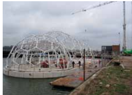
Figure 2.13: Floating Pavilion under construction in Rotterdam, The Netherlands (Deltasync, 2010).
